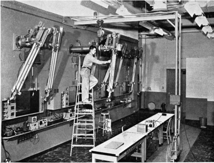
FIG. 11.—Manipulator being removed from work cell.
